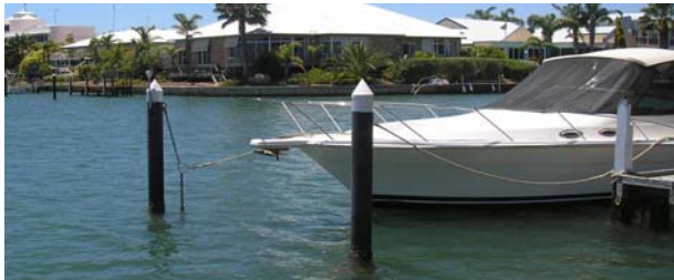
Reflective and illuminated Mooring piles
